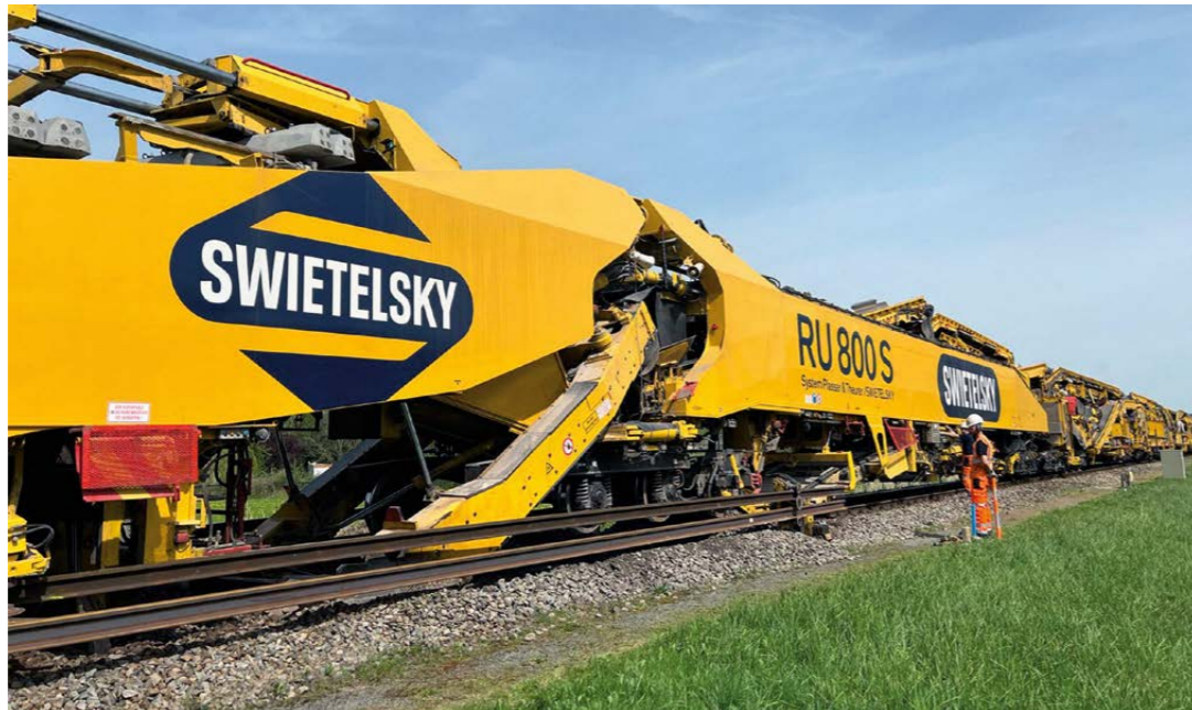
General Renovation of the Riedbahn Railway Line, Germany
