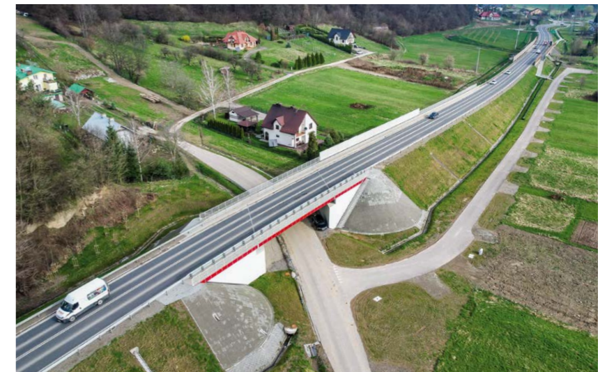
← Road No. III, Krtiny-Brezina Section, Czech Republic
