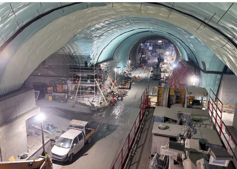
Semmering Base Tunnel, Steinhaus am Semmering, Austria
